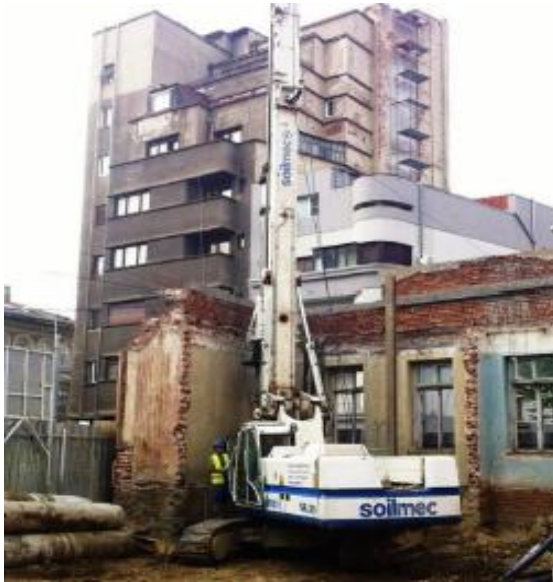
Secant piles screen near existing building \Phi 600\text{mm} 13,40m depth Tangent piles screen \Phi 600\text{mm} 13,40m depth
