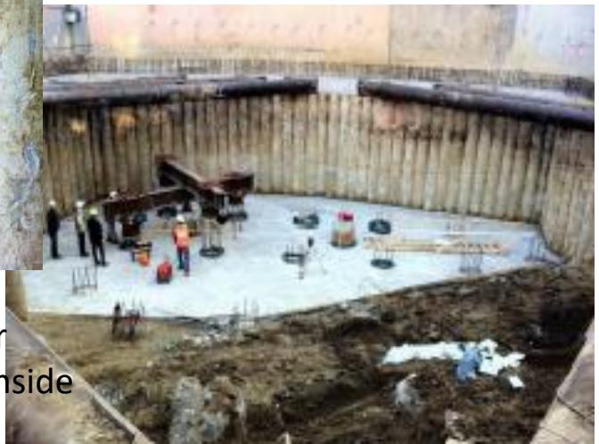
Bored piles \Phi 800\text{mm} @ 17,00m depth
