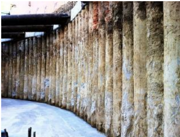
Drilling mud has been used for stabilizing the water up-pressure inside the casing protection
