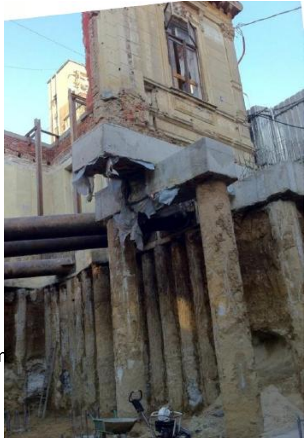
Bored piles \Phi 800\text{mm} @ 17,00m depth
